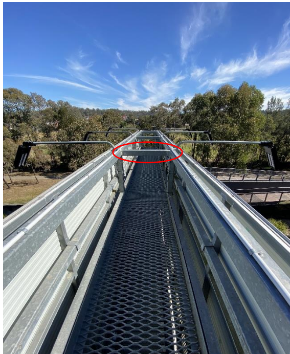
Photo 15 – Trip hazards to top catwalk (circled).
