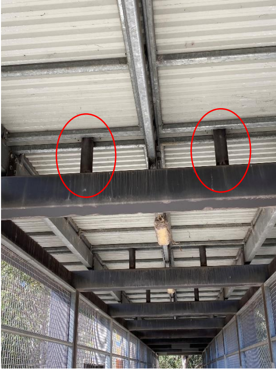
Photo 1 – Signage structure legs welded to bridge superstructure (circled).
