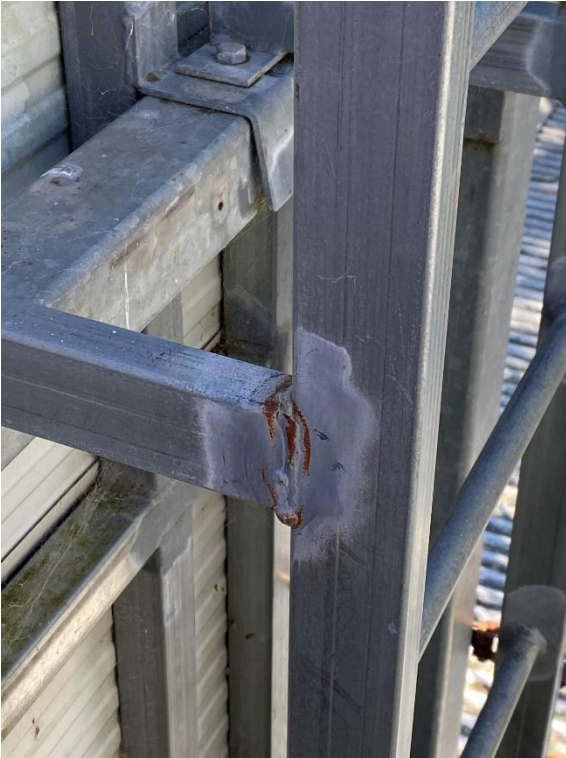
Photo 12 – Minor surface corrosion to vertical ladder support framing.
