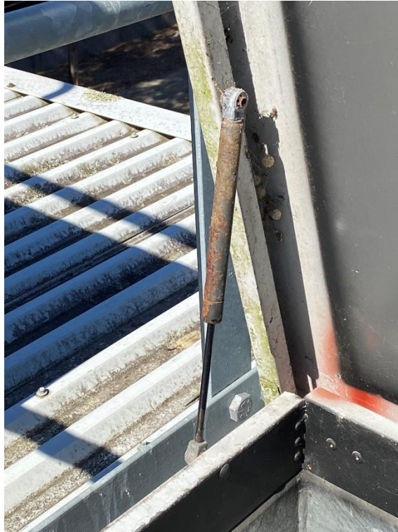
Photo 14 – Deteriorating hatch strut.
