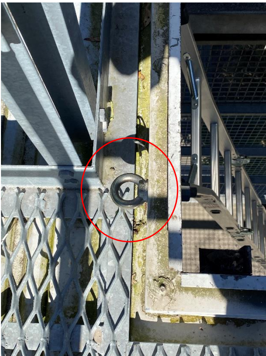
Photo 4 – Lanyard attachment eyebolt (circled)
