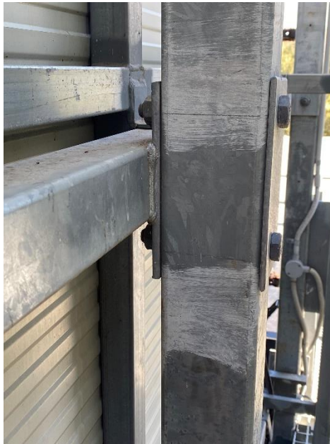
Photo 9 – Typical horizontal rail connection
